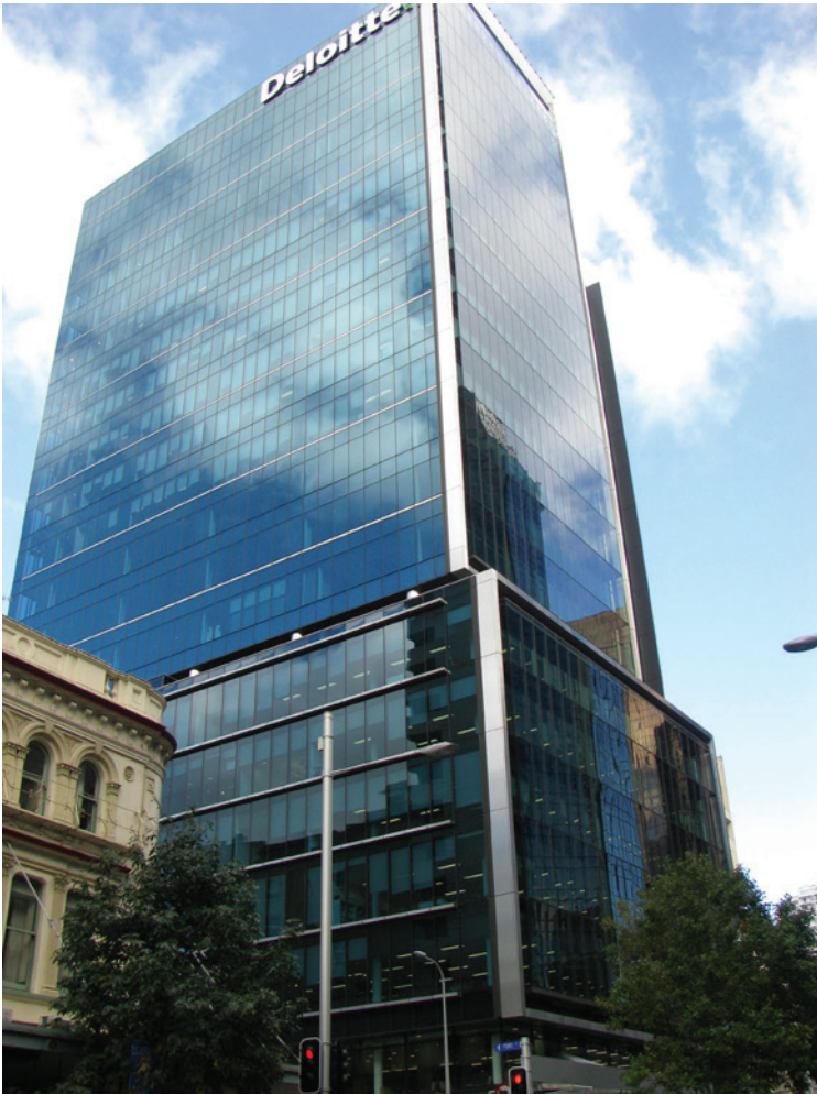
Photograph: Deloitte Centre 80 Queen Street, Auckland Built with ComFlor® 80 19 storey plus 4 basement carpark levels. 30000 sqm.
